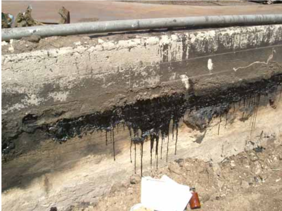
Hydrocarbon Staining adjacent to TP49
